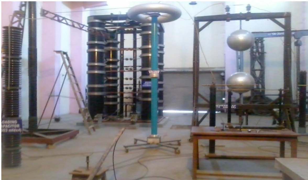
Fig.3 1.6 Million impulse voltage lab of JEC, Jabalpur, where the test at insulator under contamination level performed
